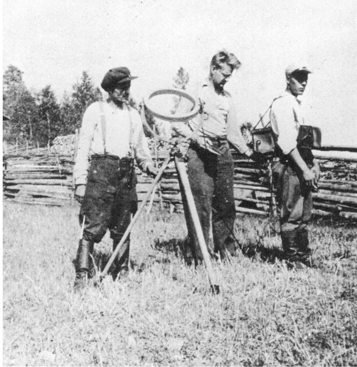
Fig. 8. Electromagnetic measurements using the intensity method (Ketola, 1986; courtesy: M. Ketola).
